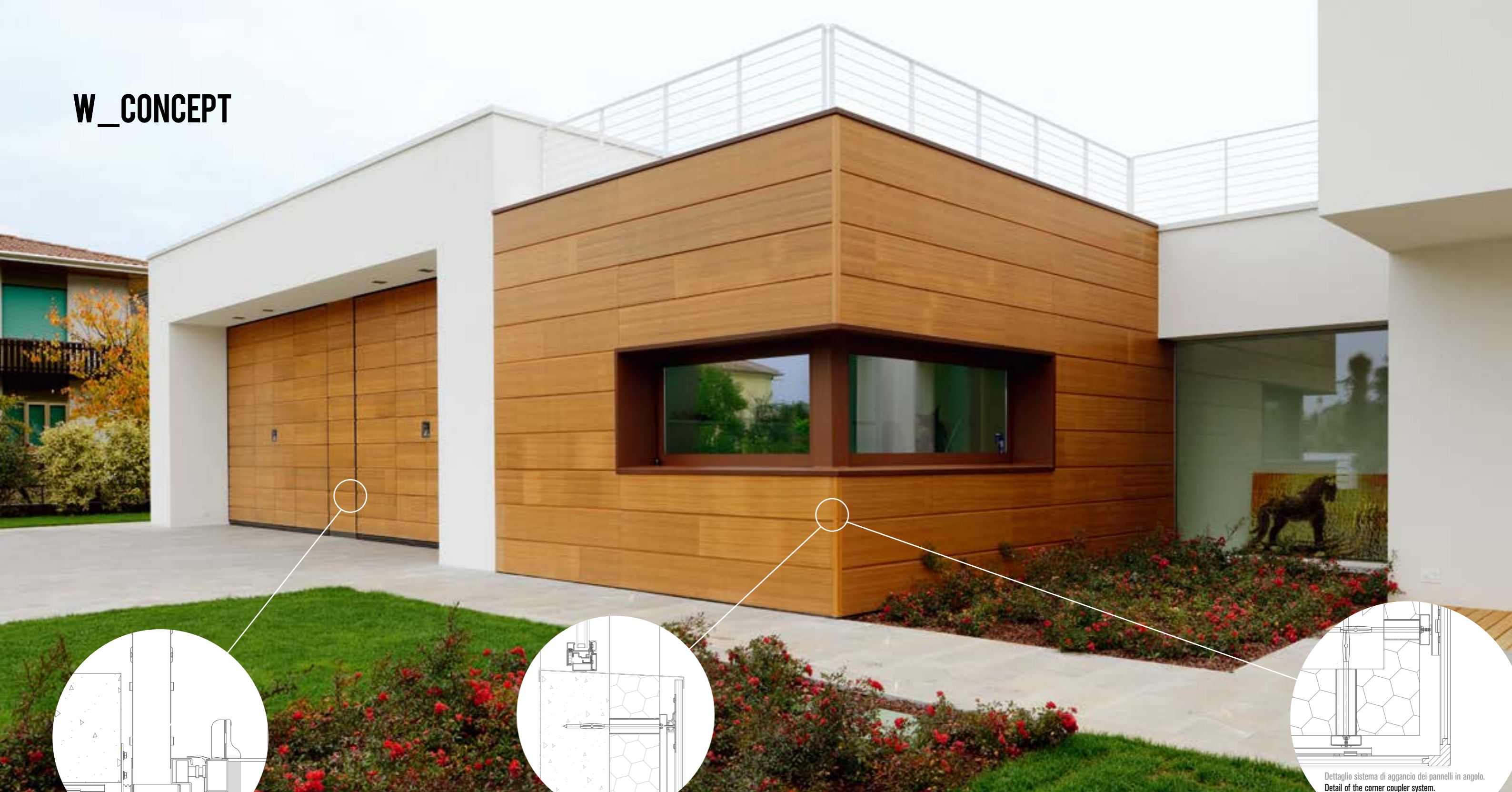
Dettaglio coplanarietà del battente porta per garage e rivestimento W_Concept. Co planarity of garage door leaf and W concept covering detail.
